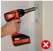
Fasteners must be installed perpendicular to the surface of the component
